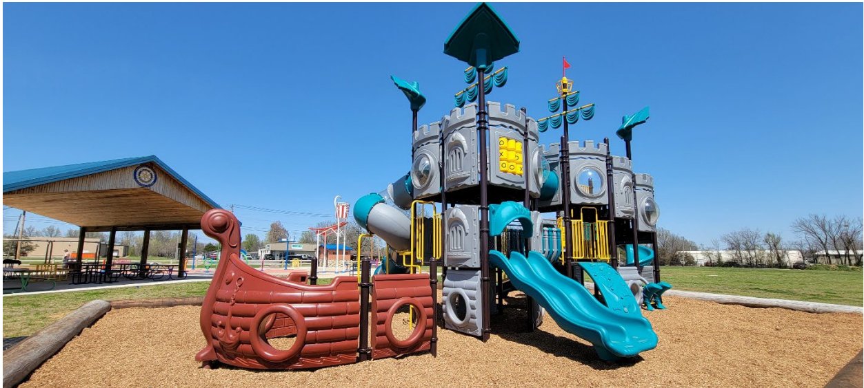
Pirate Playground Equipment Installed At The Splash Pad
