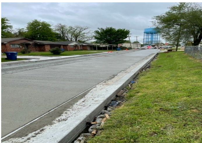
Completing Street, Curb, and Gutter Work
